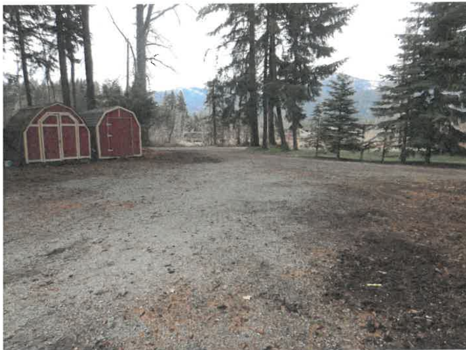
Photograph 2. Location of the potential mapped surface channel and building site; looking south. No channel is present.
